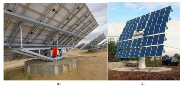
Figure 1. Classification of sun trackers according to the movement they perform (turning axes are highlighted). (a) Polar-mount sun-tracker; (b) Horizontal-axis sun-tracker; (c) Azimuth sun-tracker; (d) Dual-axis sun-tracker (polar-mount).
