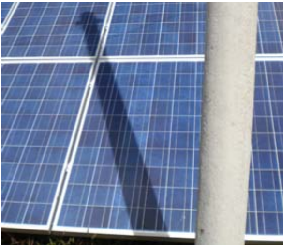
Figure 6. Wire pole shadows on the PV module.
