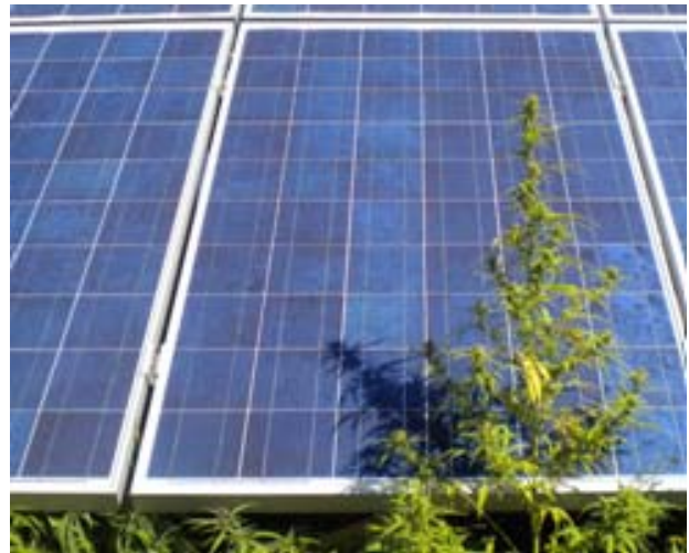
Figure 3. Plant shadows on the PV module.
