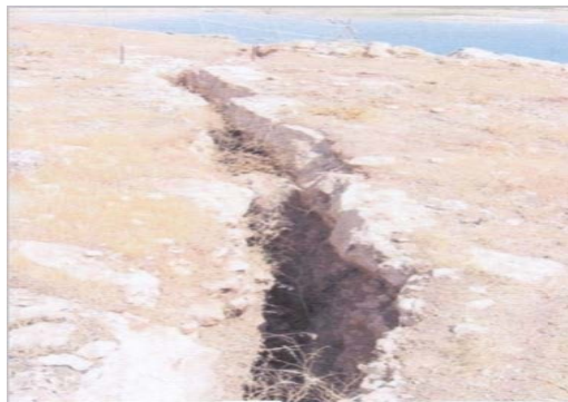
Figure 8. Ground fissure which appeared in the right abutment close to dam abutment [3].
