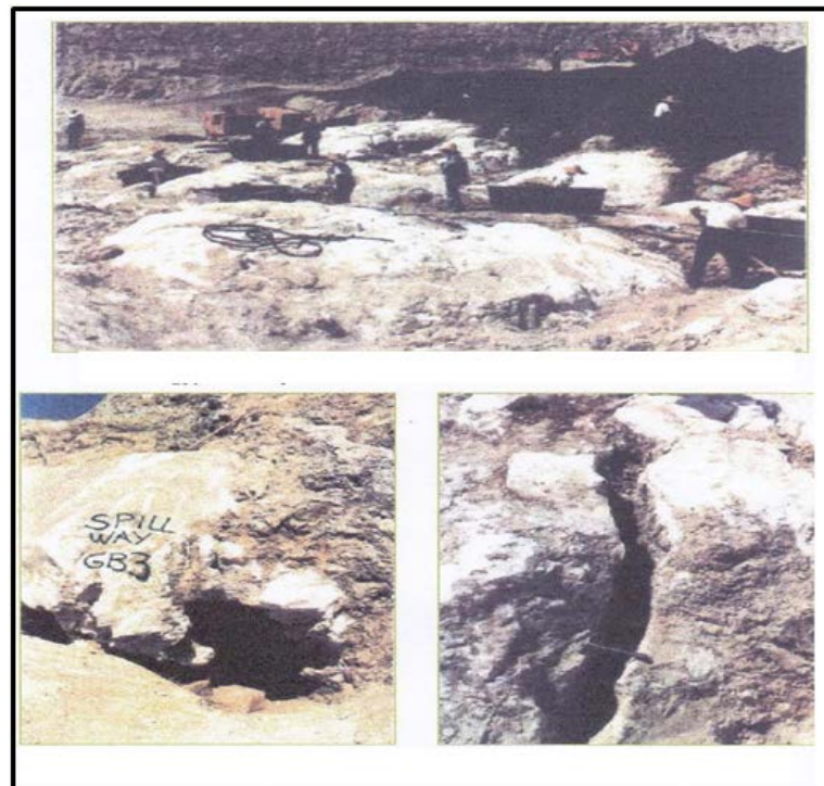
Figure 4. The badly jointed and fissured (GB3) layer found in the left bank in the foundation of the spillway chute and bucket [7].
