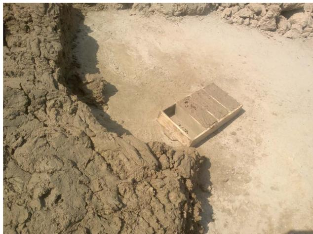
**Figure 3.** Moist clay paste prepared for casting of bricks.
