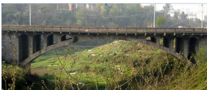
Figure 1. Foremost photo of the bridge.
