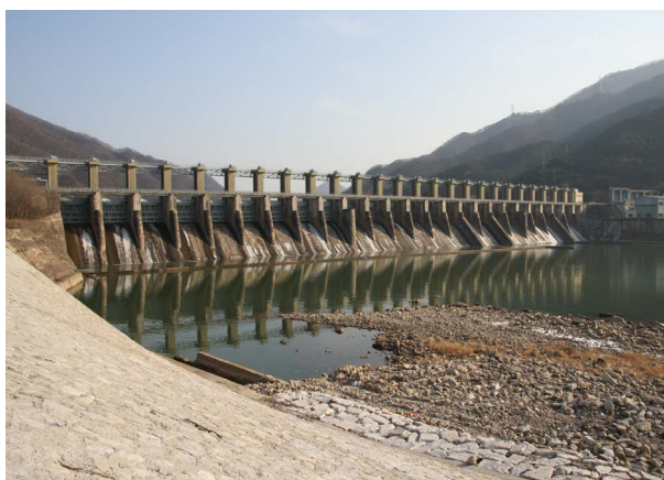
Figure 2. View of Cheongpyeong Dam.
