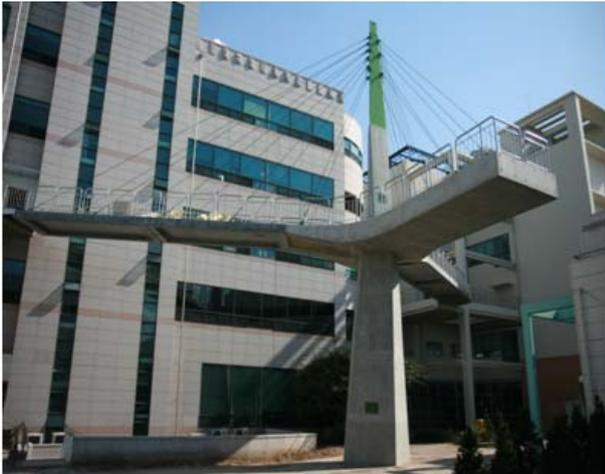
Figure 1. View of pedestrian cable-stayed bridge.
