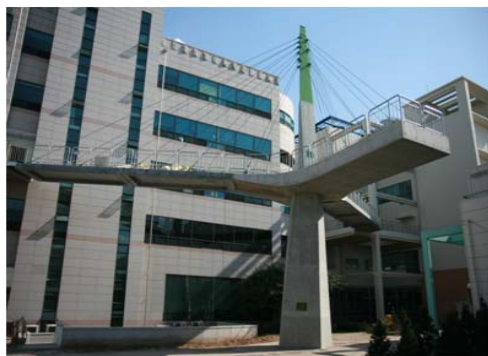
Figure 1. Super Bridge I, the UHPC cable stayed bridge at KICT.
