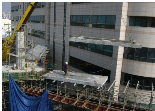
Figure 6. Installation of UHPC deck.
