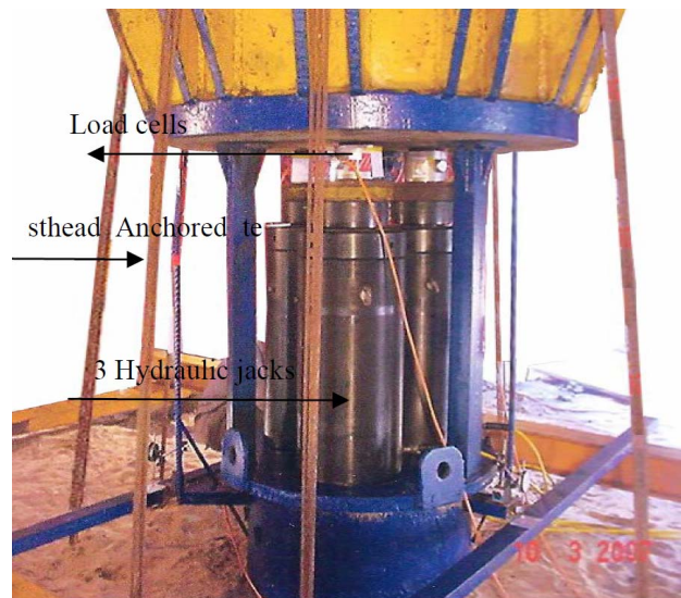
Figure 5. Pile loading setup.
