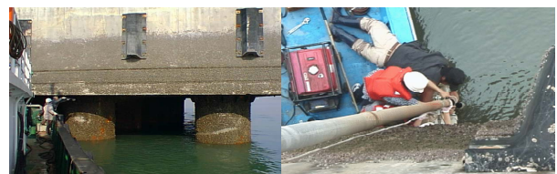
Figure 9. Pier shape of bridge and installation of scour sensor on the pier.
