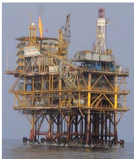
Figure 4. W11-4 jacket platform
