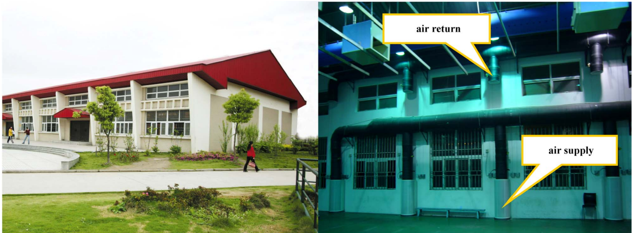
Figure 1. Outward appearance and inward mechanical ventilation of the experimental building.
