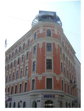
**Figure 5.** 19<sup>th</sup>-Century Apartment House: renovated and expanded attic (copyright D. Schoenbichler).
