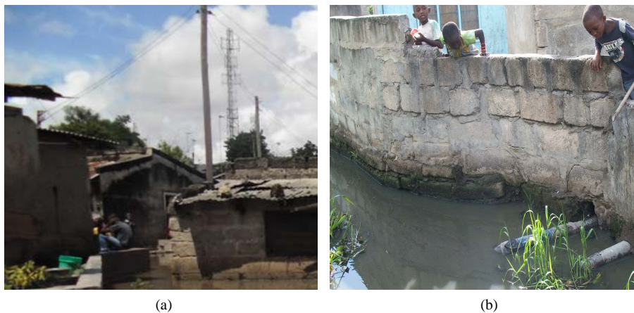
Figure 1. Sanitation conditions in Keko Machungwa. (a) A flooded toilet; (b) Pipes from a pit-latrine directed to a stream.
