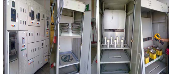
Figure 4. 3-phase electrical module of purely resistive, capacitive and inductive load.
