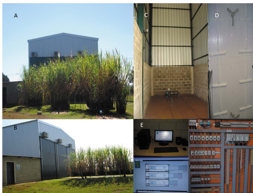
Figure 1. Photoperiod facility. A—External view with the mobile wagons; B—Photoperiod chambers; C—Internal chamber; D—Light structure in the ceiling; E—Automation Software; F—Automation panel.
