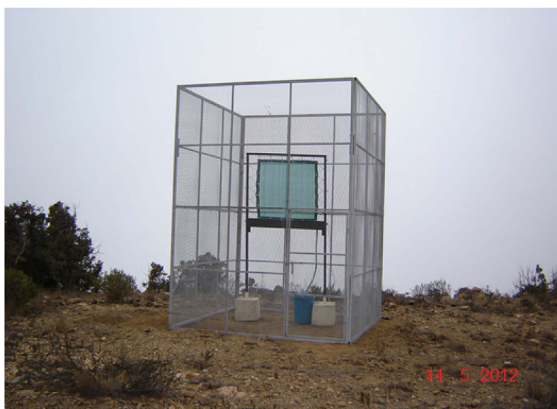
Figure 5. Fog water collection system (SFC) at Al-sooda, Assir region, Saudi Arabia.
