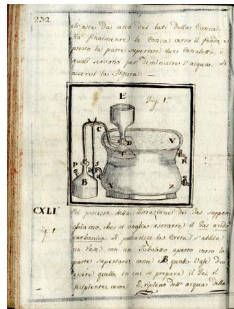
**Figure 21.** Silio's lecture course transcribed and drawn in 1819 by *E. Taranto Rosso*. Drawing of a pneumatic-chemical apparatus for extracting gases. By Courtesy of Municipal Library *E. Taranto* in Caltagirone.
