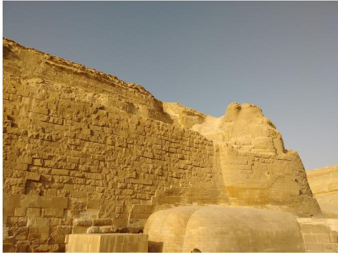
**Figure 13.** The repaired (beginning with Baraize, circa 1926) major fissure through the left waist of the Sphinx as seen from the north. Photo by M.S., June 2019.
