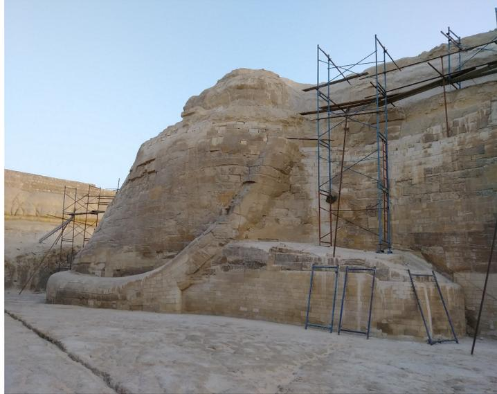
**Figure 11.** The repaired major fissure on the south side of the Great Sphinx's waist can be seen to course through the hind paw and on through the ditch. Photo by M.S., June 2019.
