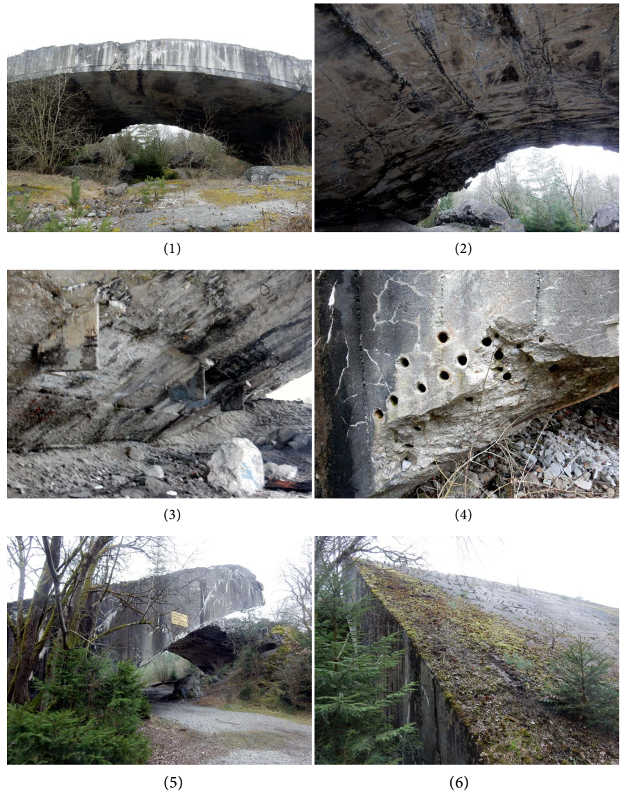
Figure 6. Weingut I—7 th arch : (1) coverage rear side with 30 cm and 5 m concrete layers, in the foreground 6 th arch coverage; (2) coverage with constructive segments; (3) coverage with constructive segments and aligned vertical protrusions; (4) dynamite holes on the rear side; (5) rear side with empty space of the fallen part and attached part; (6) coverage with aligned armour iron extremities.
