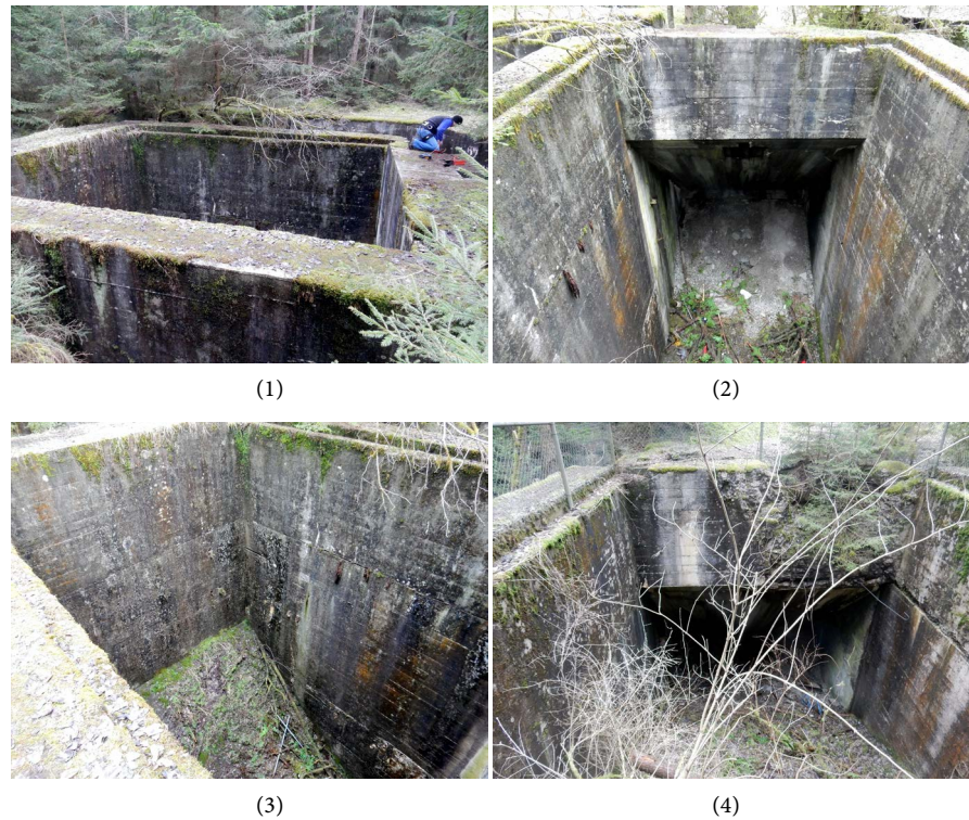
Figure 9. Weingut I —(1) first air intake/exhaust, square internal wall; (2) well entrance toward Weingut I ; (3) well inclined floor; (4) second air intake/exhaust.
