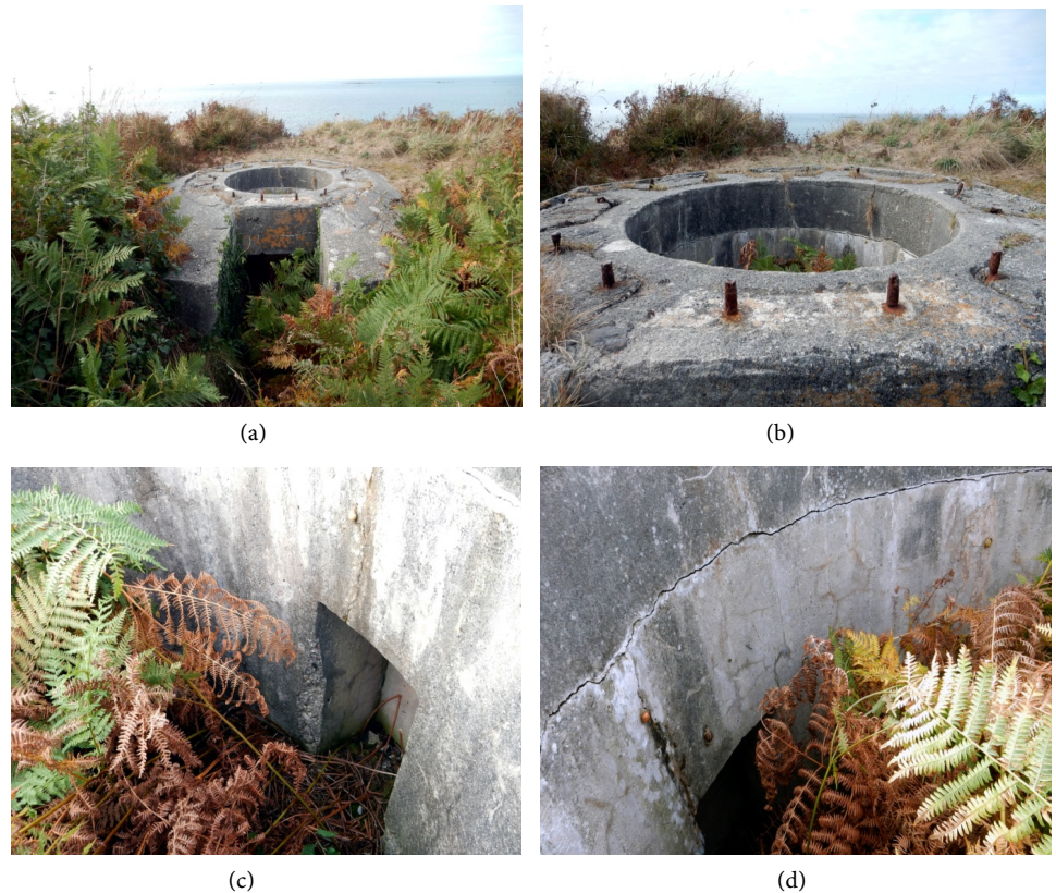
Figure 16. Vougo-Kerizoc St.P. AV 24 radar base—(a) small gun bunker with circular aperture on the couverture and small entrance to a circular room, in the foreground, barely visible, neighboring reefs (b) circularly disposed gun support joints; (c)-(d) internal circular room with ammunition niches.
