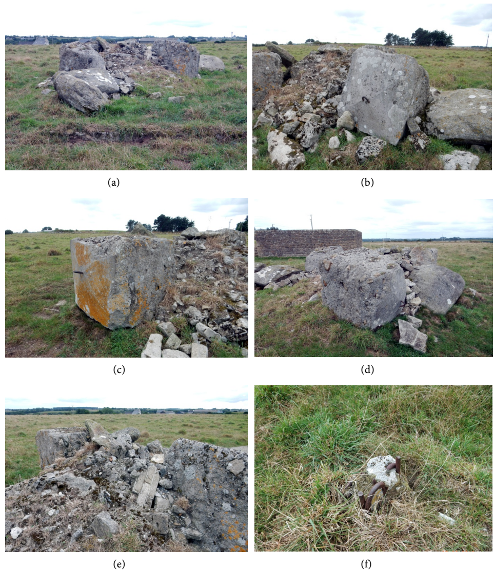
Figure 8. Kervingam-Kerdené radar base—(a) heap of stones; (b) crumbled support structure and first concrete, cubic anchoring block; (c) second concrete, cubic anchoring block; (d) third concrete, cubic anchoring block; (e) crumbled antenna support; (f) anchoring joint in the terrain.
