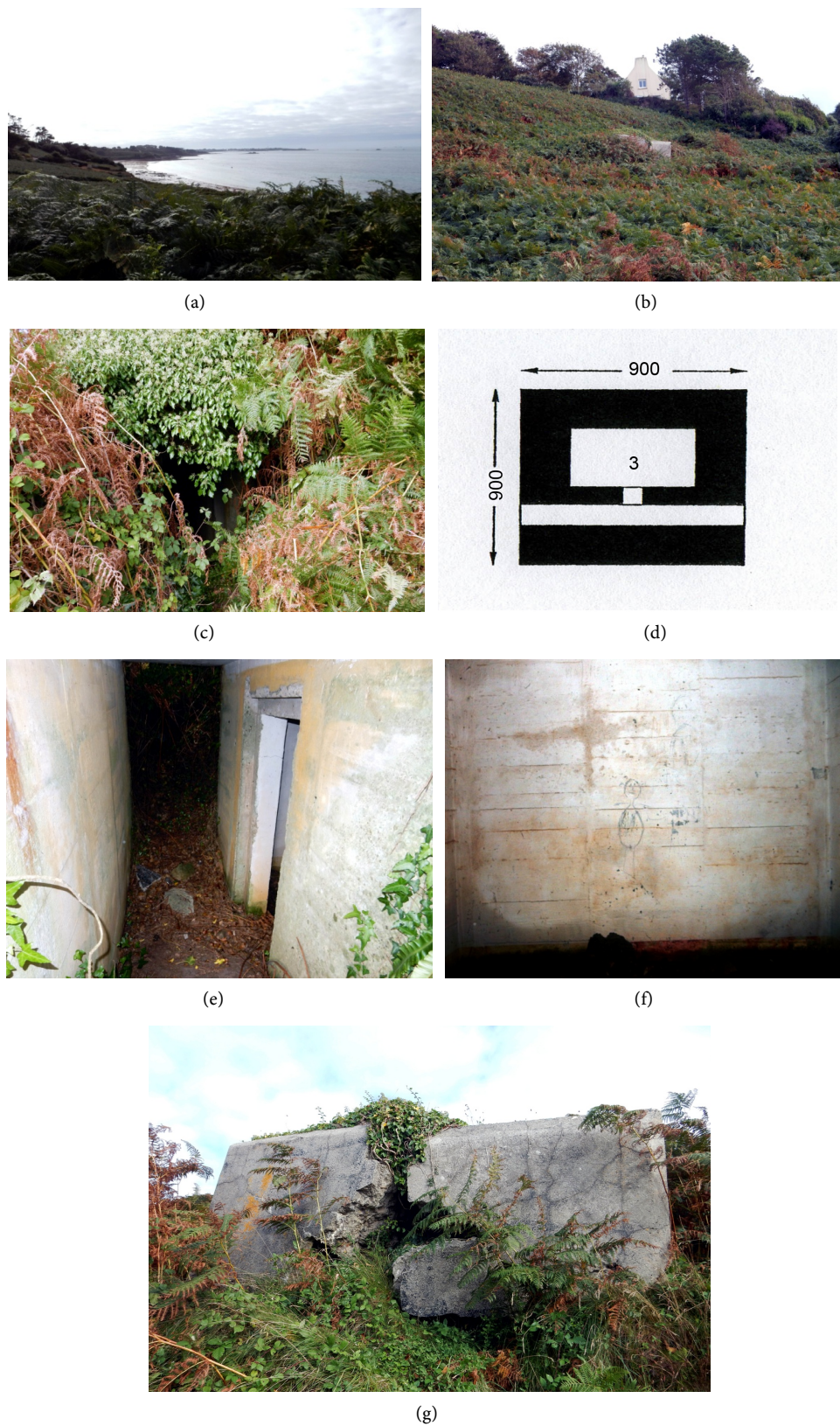
Figure 15. Vougo-Kerizoc St.P. AV 24 radar base—(a) coastal line; (b) inaccessible bunker encircled by vegetation; (c) hole in the vegetation masking one of the corridor entrances of a bunker type R702; (d) R702 plant: 3. crew room; (e) R702 corridor and room entrance; (f) R702 room preserving its original white painting; (g) dynamited small bunker.
