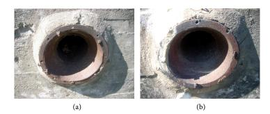
Figure 37. Hôpital des Rosais base—first aid R118 bunker, air vents of the bunker without protection grid.
