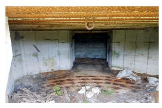
**Figure 13.** Kullak battery: R669 (c) fire room—at the centre walled rear side aperture, on the left entrance of the ammunition room, on the right entrance of the combat gas extraction system room, on the metal ceiling two joints for the gun lifting, on the floor arcuate rails of the vibration dampening system, on the left and on the right wall rests of the supports for the panels of the thermal and/or acoustic insulation system, on the floor arcuate rails of the vibration dampening system.
