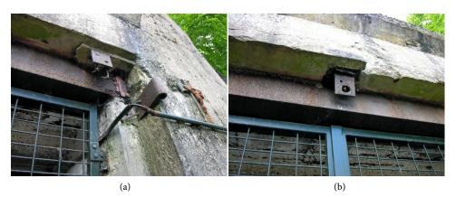
**Figure 32.** Les Ormeaux battery: (a), (b) R669—details of the original doorposts of the fire room front aperture.
