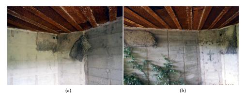
**Figure 7.** Kullak battery: (a), (b) R669 (b) interior of the fire room with panels of the thermal and/or acoustic insulation system on the walls.
