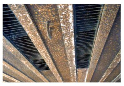
**Figure 9.** Kullak battery : R669 (b)—fire room ceiling, grids of the combat gas extraction system and one of the two joints for the gun lifting.
