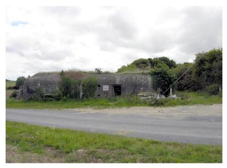
**Figure 22.** Ville Besnard logistic base: lonely bunker—on the left front aperture of the fire room, at the road level, on the centre four air vents, on the right personnel entrance, behind the bunker, cistern area (a2).
