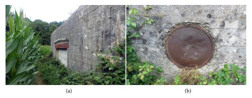
Figure 12. Kullak battery: (a) R669 (c)—walled rear side aperture; (b) R669 (c)—grid on the exhausted combat gas pipe.
