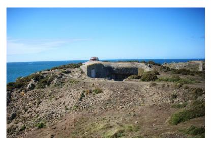
Figure 16. Pointe de la Varde support point: R120a observatory bunker (48°40'53.4"N, 1°59' 23.4"W)-on the left, white painted, entrance of the uncovered lookout post and the observatory bell, in the middle bunker entrance and close combat room, on the right protective wing.
