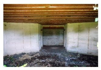
Figure 5. Kullak battery: R669 (a) fire room—at the centre walled rear side aperture, on the left entrance of the ammunition room, on the right entrance of the combat gas extraction system room, on the metal ceiling distorted joint for the gun lifting.
