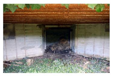
**Figure 8.** Kullak battery: R669 (b) fire room—at the centre walled rear side aperture, on the left entrance of the ammunition room, on the right entrance of the combat gas extraction system room, on the metal ceiling two joints for the gun lifting, on the left and right walls panels of the thermal or acoustic insulation system.
