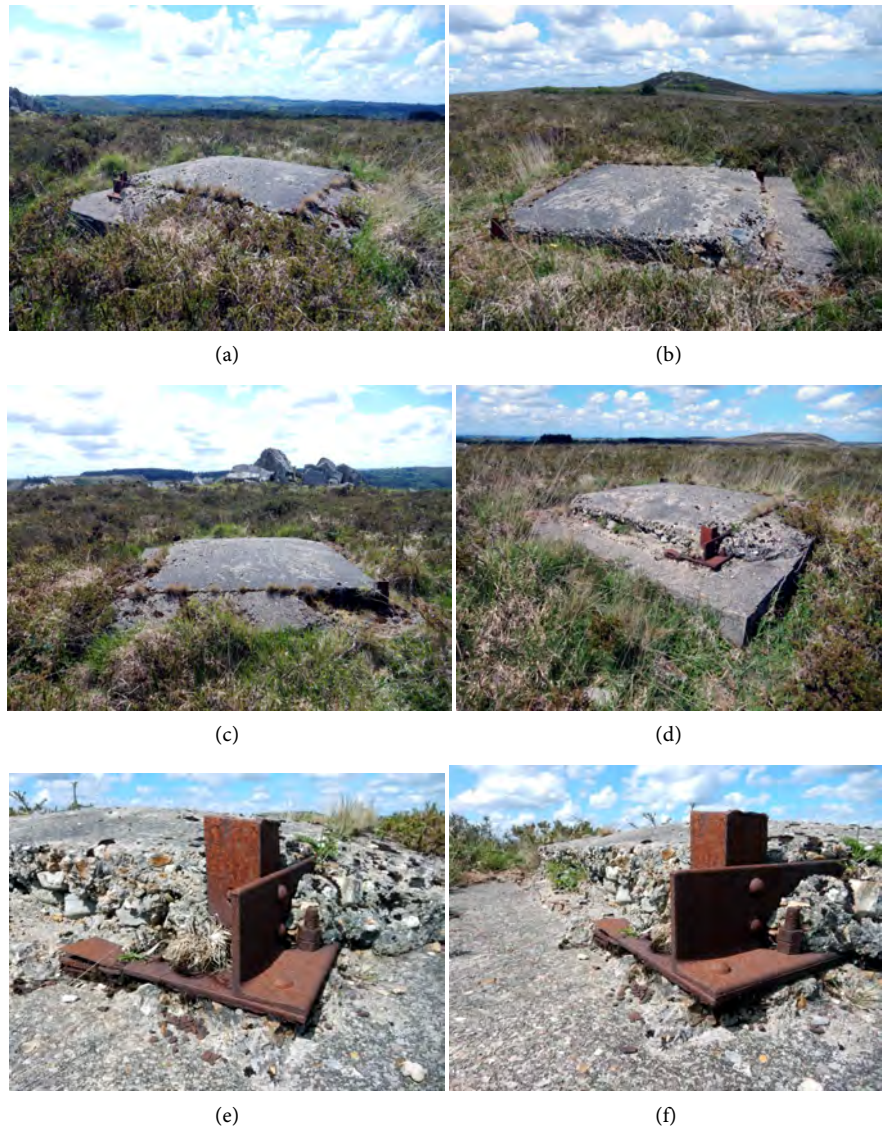
Figure 4. Mast vestiges—(a) Mast support, north vision; (b) Mast support, east vision, on the background the 17 th cen. Saint Michel chapel (n) on Mont Saint Michel de Brasparts; (c) Mast support, south vision, on the background group of basaltic blocks emerging from the terrain; (d) Mast support, west vision; (e) Mast fixing structure, thick concrete layer with EroVili pebbles; (f) Mast fixing structure, rivets and fixing bolt.
