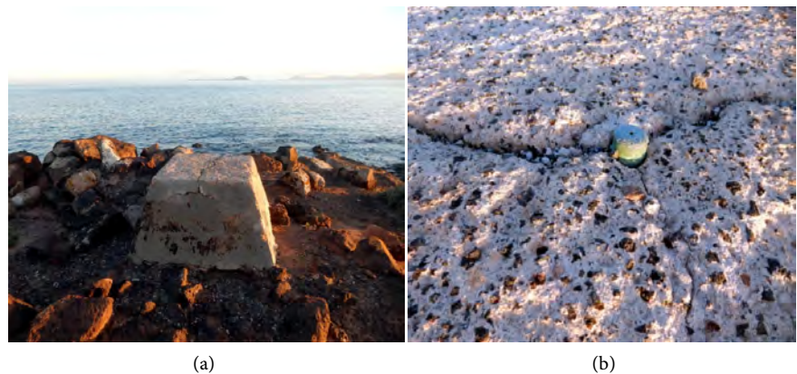
Figure 4. Truncated, pyramidal base (3)—(a) General view, on the foreground, Lobos island in the middle and Fuerteventura island on the right; (b) Local, small magmatic pebbles mixed with concrete and cylindrical, metallic shaft at the centre of the square top surface.
