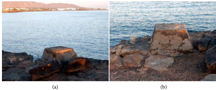
Figure 3. Truncated, pyramidal base (2)—(a) General view, on the foreground Playa Blanca; (b) Thin concrete layer covering portions of the side surfaces.
