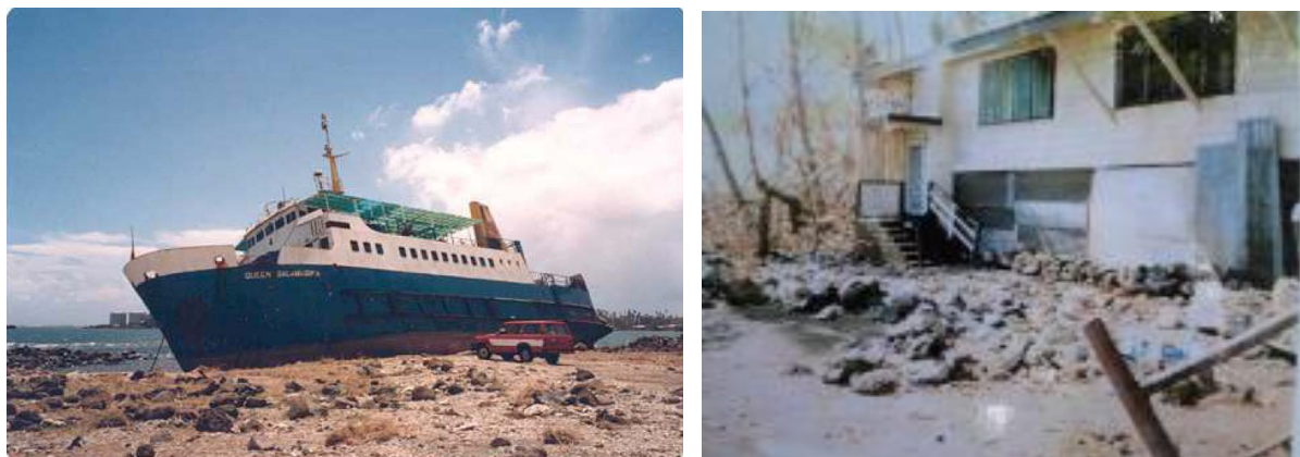
Figure 9. Damage in Apia caused by category 4 tropical cyclone Ofa : The beaching of the passenger/cargo ferry Queen Salamasina in Apia (left) and damage to houses (right).
