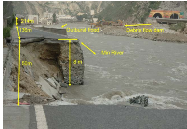
Figure 8. Outburst flood of dammed lake induced by Qipan Gully destroyed Dujiangyan-Wenchuan Highway at the outlet.
