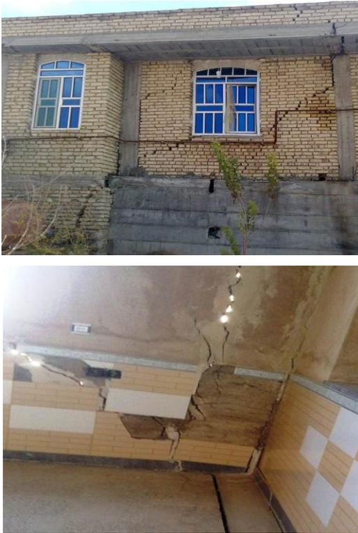
**Figure 11. The created cracks inside and outside of the building due to land subsidence.**
