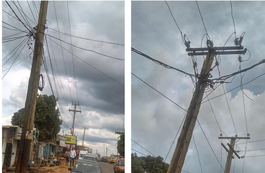
**Picture 1.** State of the supports of line (TEG picture).
