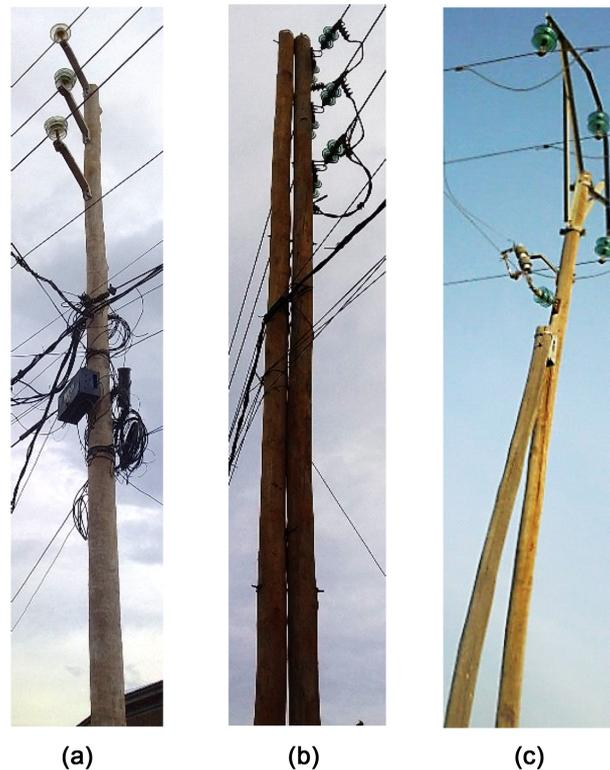
**Figure 2.** Types of poles according to the assembly mode.
