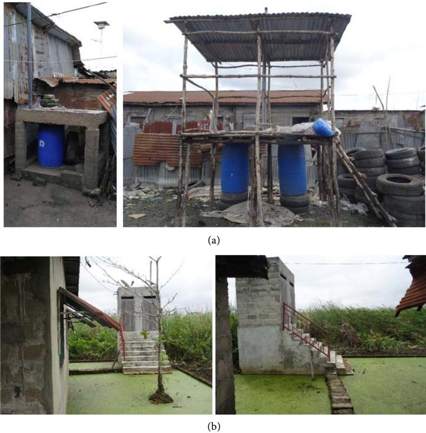
**Figure 4.** Experimental septic tanks in plastic polyethylene at Ahouansori Towéta (a) and ecological above-ground watertight pit latrine in swampy environment of Agla in Cotonou (b) (Photos: H.S. Totin Vodounon, August 2019).
