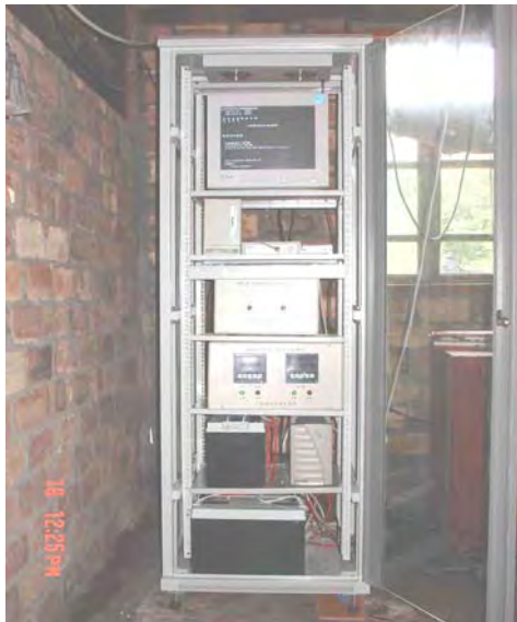
Fig. 5 Field data collection & monitoring station
