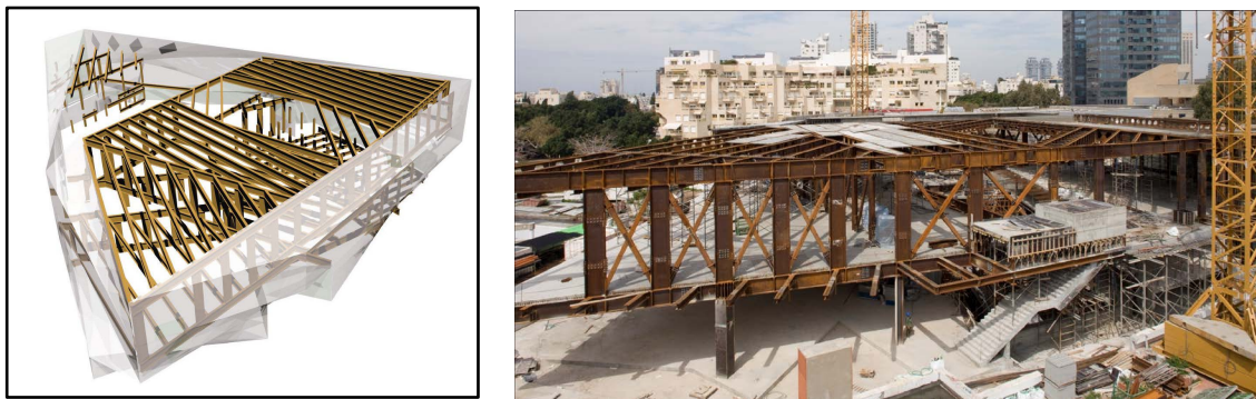
Figure 5. Structural scheme of building, left. Assembly of Vierendeel trusses, right.
