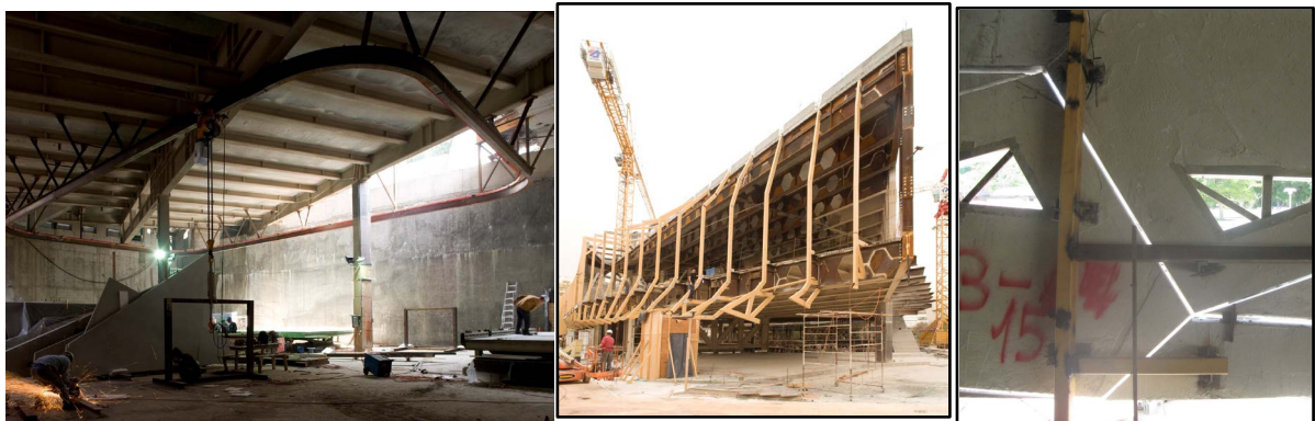
Figure 7. Assembly of façade. Left: tilting casting table and rail suspended from ceiling for manufacturing the panels in the basement. Middle: auxiliary frame at two meter intervals; Right: backside of panels welded to the frame prior to sealing.
