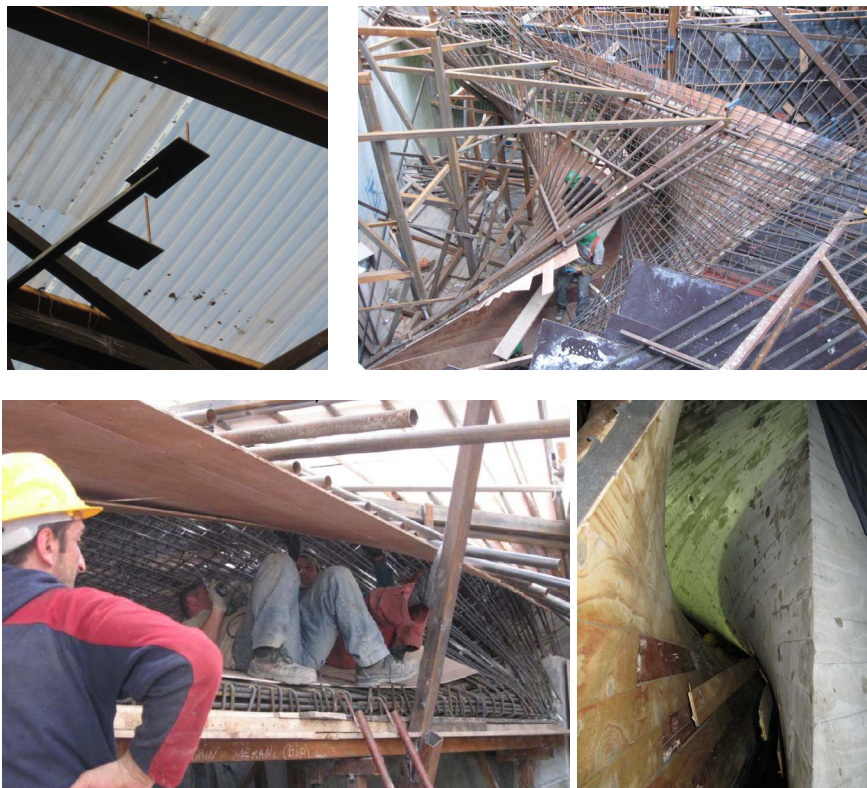
Figure 6. Construction of lightfall. Top: welded reference point for hypar, left; metal pipes for bracing formwork, right. Bottom: workers adjusting formwork, left; concrete after removal of formwork, right.
