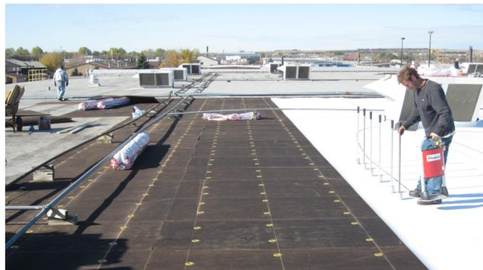
**Figure 7.** Attachment of a thermoplastic single ply membrane using inductively heated plates. The installer is holding the heating machine, while placing weighted magnets onto the membrane above plates that have been heated. The magnets apply pressure between the plates and the membrane to promote fusing of the two.
