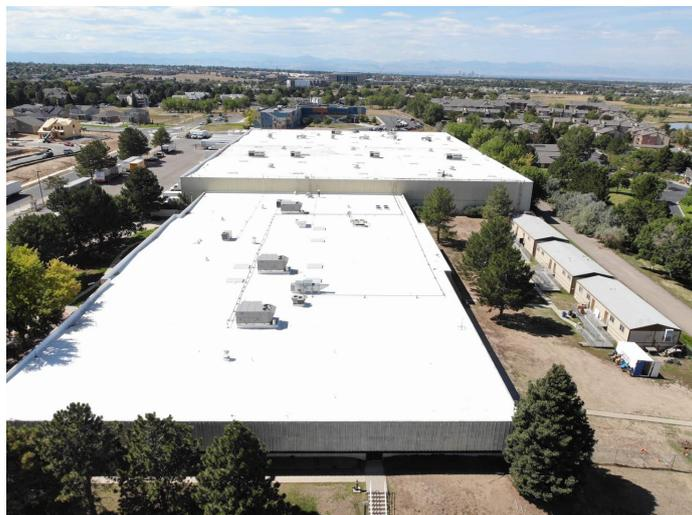
**Figure 6.** Examples of big box construction, with a reflective roof membrane (Image courtesy of R & R construction, LLC, Denver, CO).
