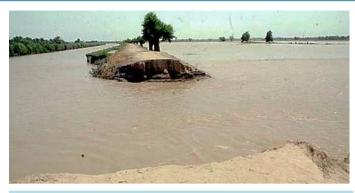
Figure 2. View of breach along Mir Wah Canal, Sindh [11].
