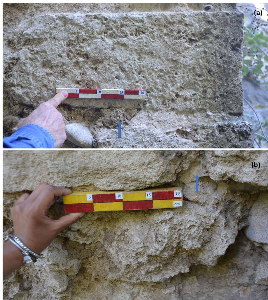
**Figure 10.** The phytoclastic travertine ashlars, showing the characteristic pores, and the mortar of arch 2 (a) and arch 3 (b), from which the samples PO 1 and PO 9, PO 2 and PO 10 were collected, respectively. The mortar is highlighted by arrow.
