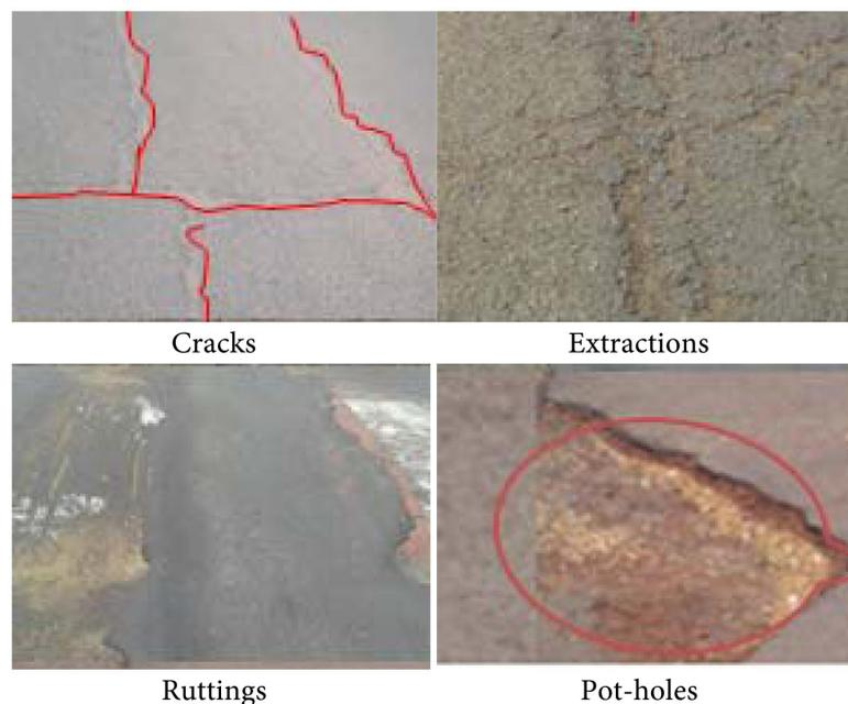
**Figure 1.** State of road degradation in Senegal.
