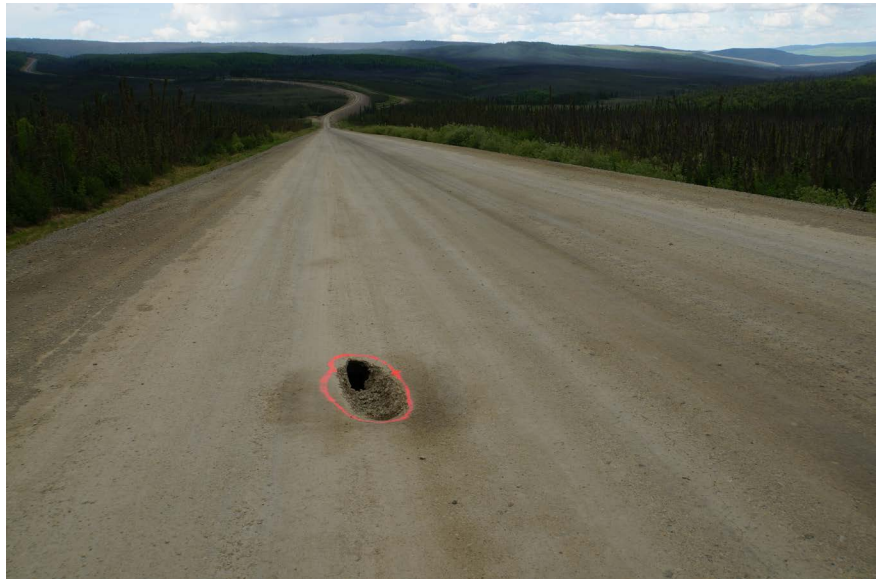
Figure 36. The Dalton Highway which has pink markings to warn drivers that there are sink holes where the permafrost has melted under the road bed. Photograph by Lois Wright Morton.
