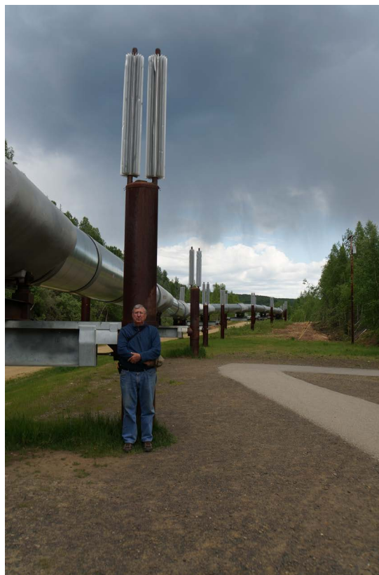
Figure 35. Heated pipes built into vertical supports for holding up the Alaska pipeline.
