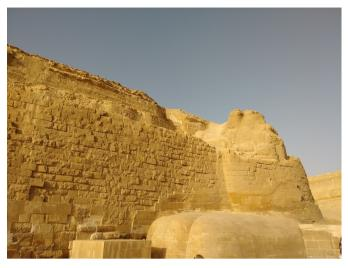
**Figure 13.** The repaired (beginning with Baraize, circa 1926) major fissure through the left waist of the Sphinx as seen from the north. Photo by M.S., June 2019.
