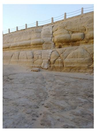
**Figure 12.** The southern extent of the major fissure through the enclosure wall viewed from the northwest along its course through the ditch floor. Modern masonry repairs have covered the fissure. Photo by M.S., June 2019.
