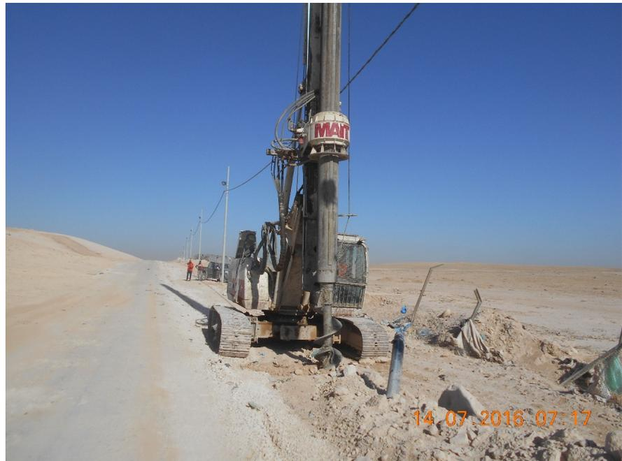
**Figure 6.** Machine used for drilling of the wella.
