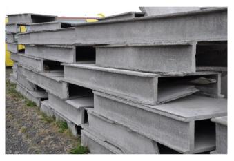
Figure 5. Faulty CBPB box elements stacked outdoors.
