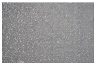
**Figure 4.** The unprotected surface of a box element in wall of the factory building (after 13 years outdoor weathering).
