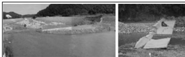
**Figure 1.** Case of weir destruction in Korea (Buk Stream and Baebong Stream).
