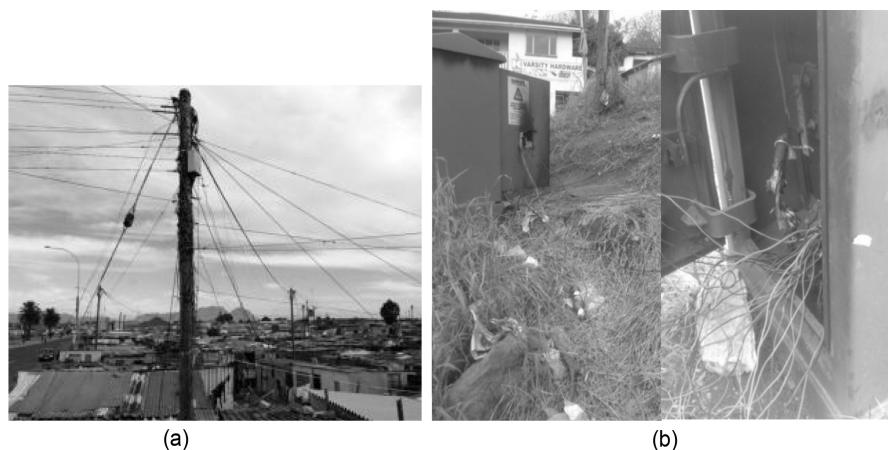
Figure 2. Illegal power connections in Durban. (a) connections to homes [7]. (b) connections from a transformer Pictures by: K. Mubiana, Durban.
