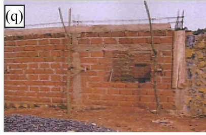
House in construction with wall in Compressed earth block-Tubah-Mezam (NW region)
