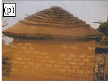
House with compressed earth block with roof with straw-Bangam-Tibati-Djerem (Adamawa region)
