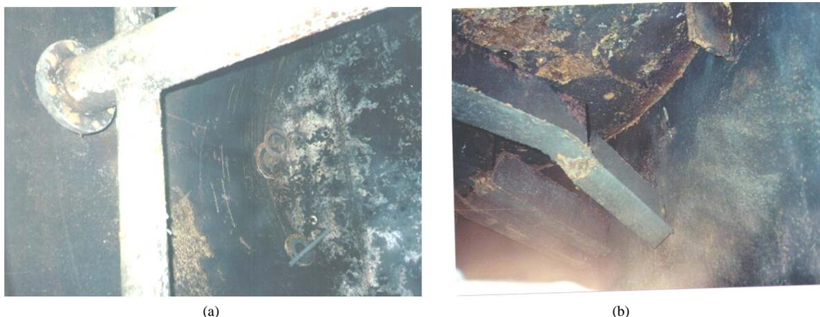
**Figure 3.** Steel tank damaged by corrosion. (a) Interior of a steel tank under analysis; (b) reinforcement of the false bottom plate. View from below the false bottom.
