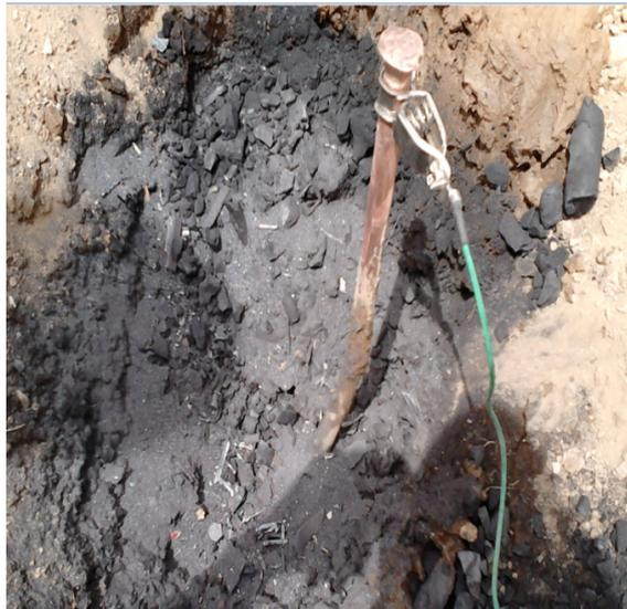
**Figure 4.** Addition of the Dead Sea water with Coal and iron-filings to the hole of grounding system.
