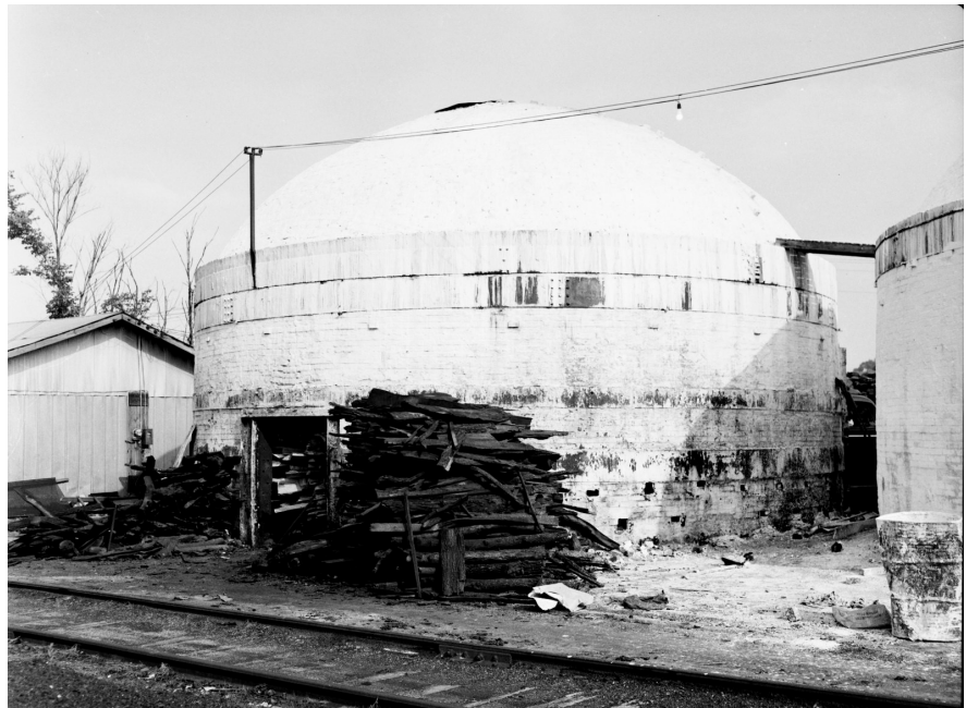
Figure 9. A circular charcoal kiln with a beehive type top, similar to the kilns along Wisconsin's rail lines. Charred slabwood piled in front of the kiln (Credit: Ohio Agricultural Experiment Station).
