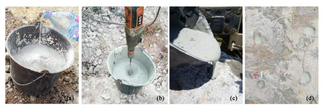
**Figure 3.** Steps of the NEEM mixture process. (a) Adding water in NEEM powder; (b) Mixing; (c) Pouring into predrilled holes; (d) Holes filled with NEEM.
