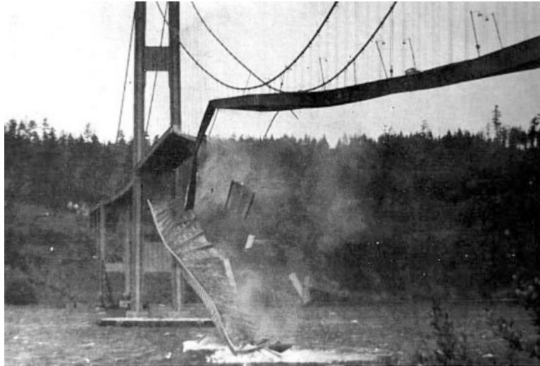
**Figure 2.** Collapse of Takoma Narrows Bridge.
