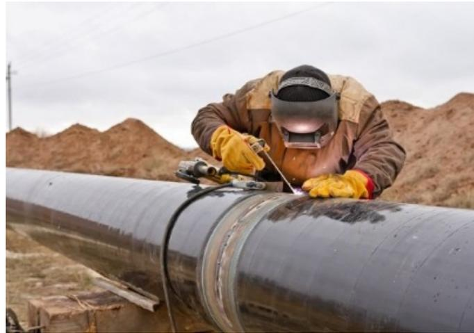
**Figure 23.** Construction site in welding pipeline.
