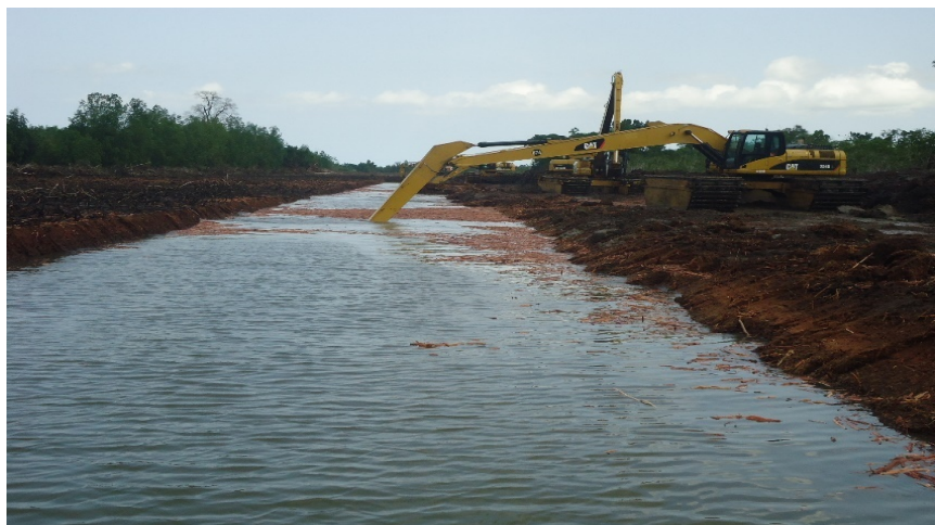
Figure 9. Finishing/leveling of ditch bottom (Source: NESTOIL [22]).
