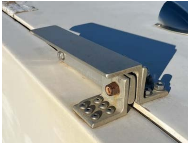
Figure 3. Photograph of a closed folding lid stay hinge.
