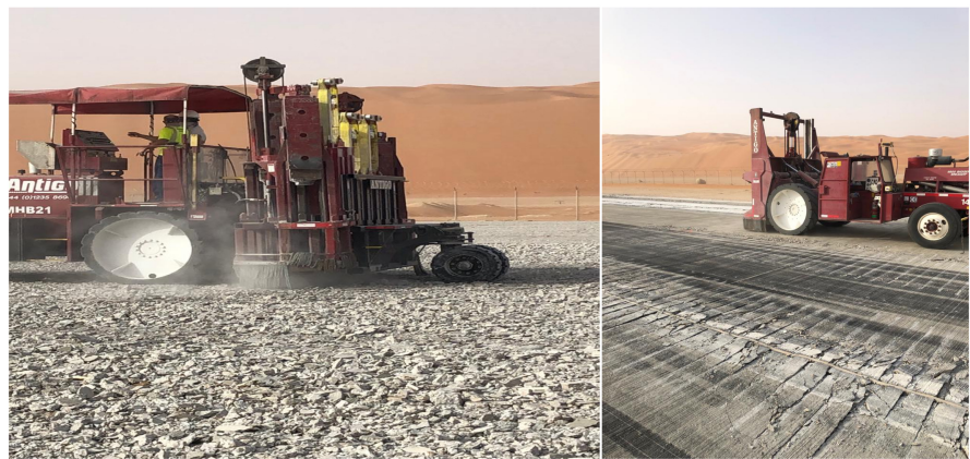
Figure 4. Antigo Construction Inc. equipment (MHB Badger Breaker on the left and 8600 Badger Breaker on the right) on operation at Shaybah Airport Runway.
