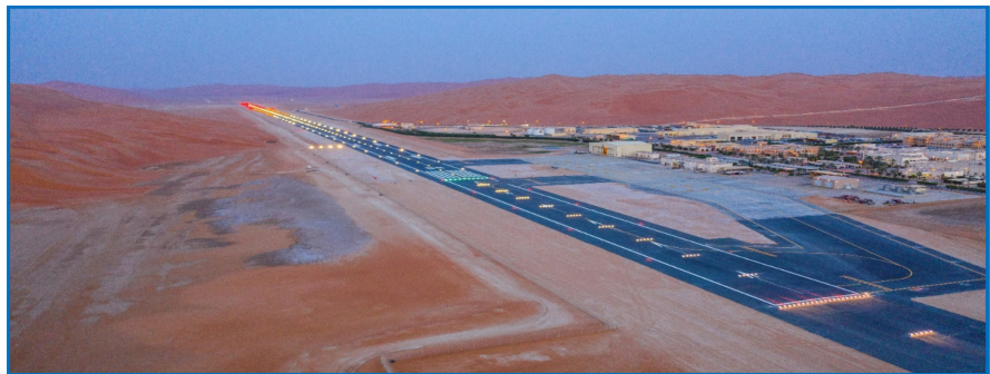
Figure 6. New Shaybah airport runway pavement after implementation of rubblization and overlay with hot mixed asphalt (HMA).
