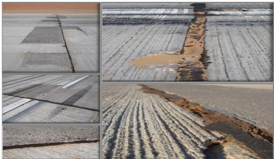
Figure 1. Deteriorated conditions of the old Shaybah Airport runway concrete pavement.
