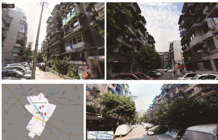
Figure 2. Current situation of old Buildings in Xiaojiahe. (Source: Author).
